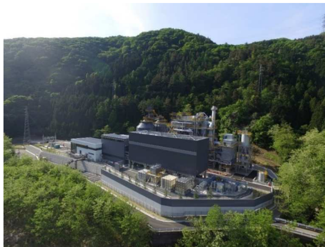
[Project 03-2 Otsuki Biomass Power Plant]
